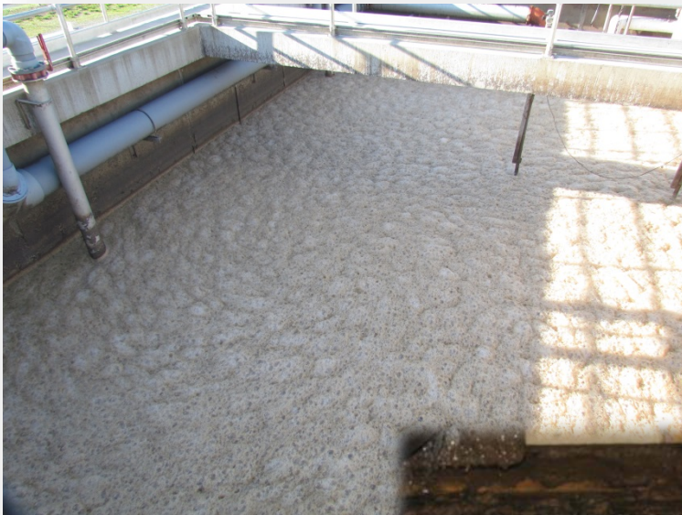
Foaming in Aeration basin, Zooglea on belt press
