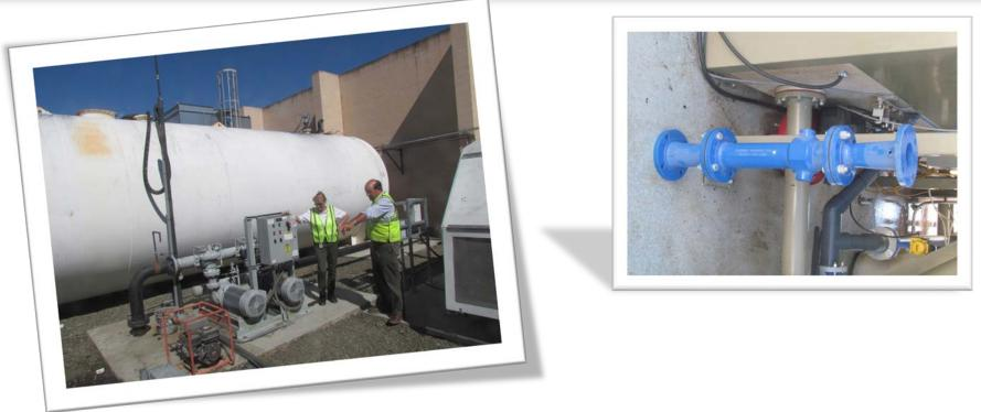
POAA is a biocide with a very long stable life in wastewater. High dosages can easily kill a small wastewater plant. Return of a small amount of RAS and bioaugmentation used upstream in EQ to help break down the biocides prior to entering the Aeration basin Venturi used to increase DO levels in the EQ
