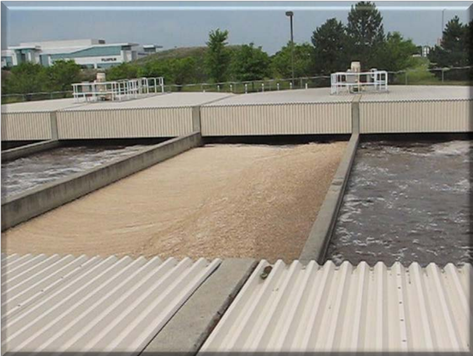
Oxidation ditch 7-7-11 Before Bioaugmentation
