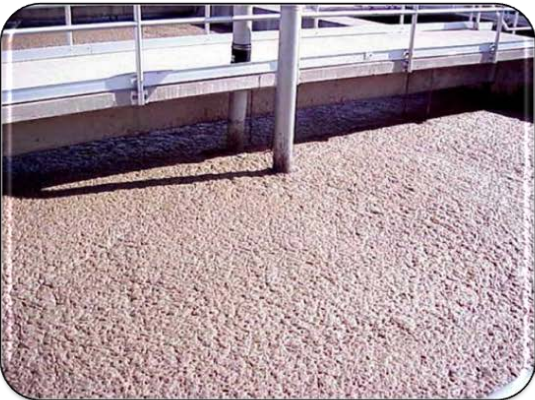
Foaming in aeration basin
