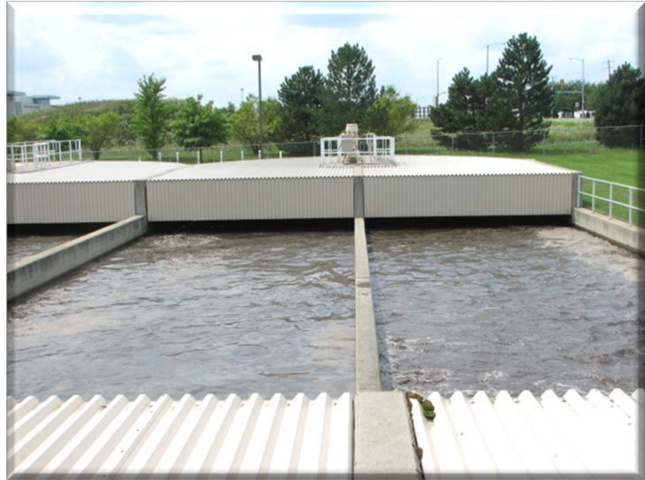
Oxidation ditch 8-8-11 After Bioaugmentation
