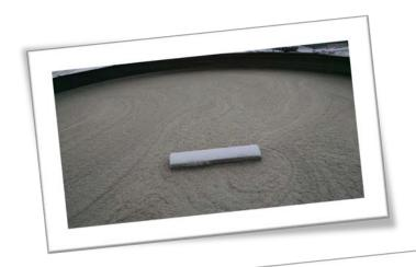
High foaming due to overload of BOD
