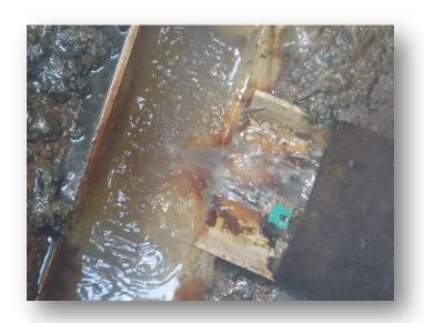
High levels of zooglea and slime in lift station due to oils and grease.
