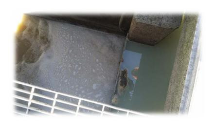
Oils from productions as well as lubricating oils causing high levels of organics
