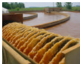
Automatic weir washers can easily help keep weirs cleaned
