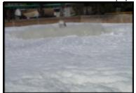
foaming. Excessive foam, especially in an aeration basin, can cause a variety of problems. A foam blanket on the aeration basin can interfere with oxygen uptake of the microorganisms and hinder BOD reduction. Foam can also cause the
