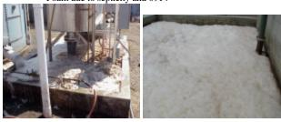
Very young sludge at a winery, spilling out of equipment -Young sludge at meat packing plant - surfactants in DAF upstream causing some of the foaming also
