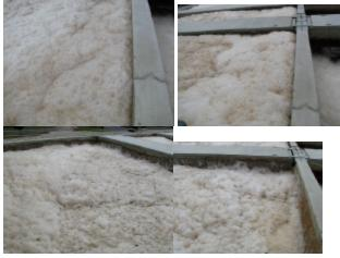
These 4 photos show a plant with serious foaming. The foam was almost up and over the edge in the top two. After topical addition of antifoam, you can see it dropped the foam 8-10 inches instantly.
