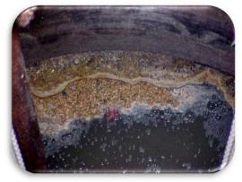
What are signs that the product is working-Foaming in the lift stationwhite foam at first shows the bugs are in a high growth phase, as the foam turns to a light brown, they are getting a little older.
