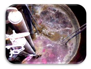
Application of product is improper here, pink product all over the top of the grease and not really in contact with the water
