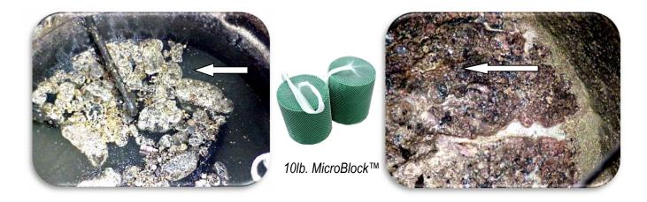
These have been called "Floating Turtles"- Hard solid formations that float around in the lift station. These can interfere with the pumps and can clog the pipes. Sometimes using a liquid product to spray on these can help reduce their size and shrink them faster.
