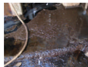
Blocked sewer with oil build-up Oil leaking off machines
