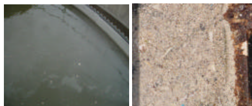
Here is grease floating on the surface of the secondary
