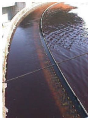
Here is a primary clarifier and this is a secondary clarifier with hydraulic overload.
