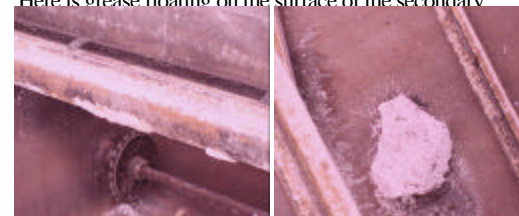
Here is grease floating on the surface of the secondary
