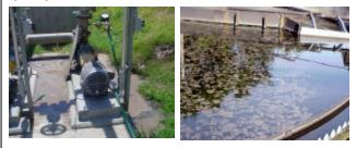
**Mechanical equipment:** Pumping, RAS lines, suction, drawdown tubes, rakes, these are all mechanical parts that must be kept in good working order in order for successful operations of the clarifier.
