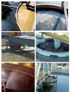
should be standardized so that all operators use it at the same time, and at the same location of the weirs. The sludge judge can be a good visual of what is going on under the surface of the clarifiers. Are you rat holing, is the bed floating, does it have black spots, what does the rag layer look like?
