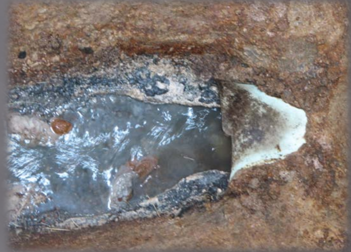
Grease in Manhole outside Chinese restaurant prior to bioaugmentation
