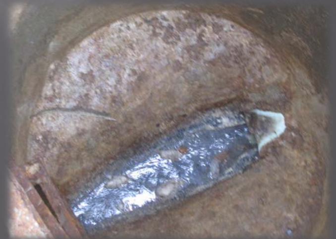
Grease in Manhole outside Chinese restaurant prior to bioaugmentation
