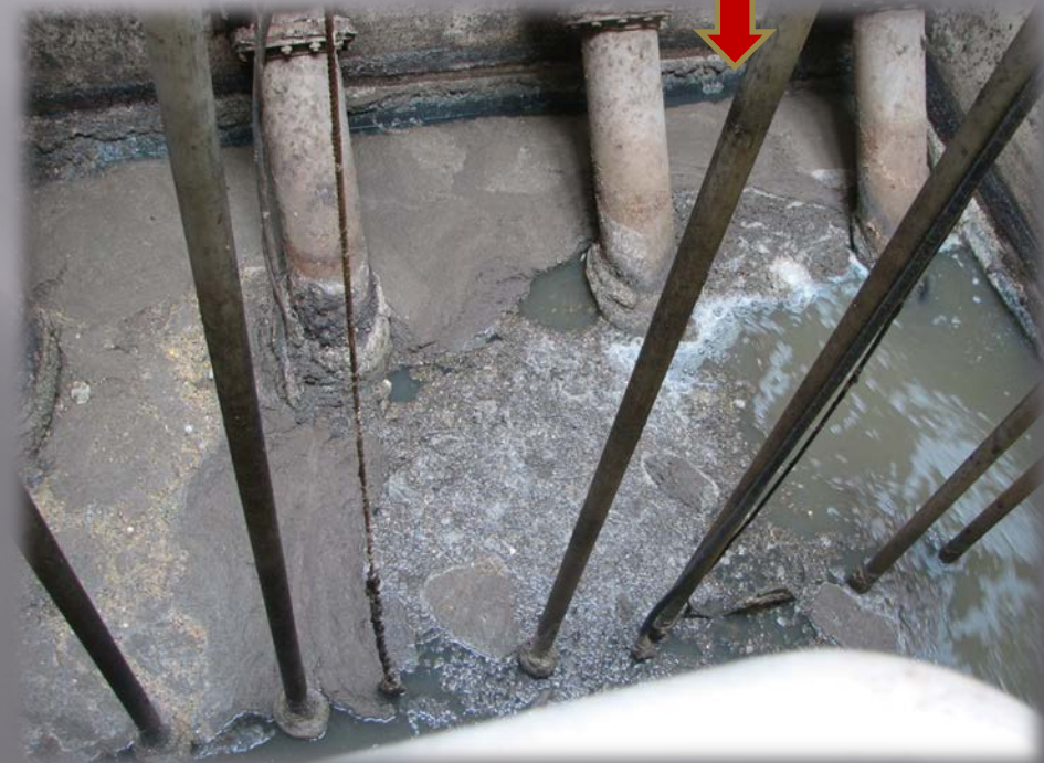
Notice the grease shelf along the walls 7-7-11
