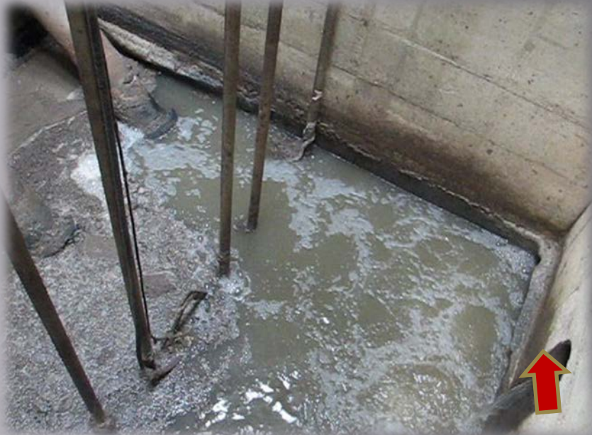
Notice the grease shelf along the walls 7-7-11
