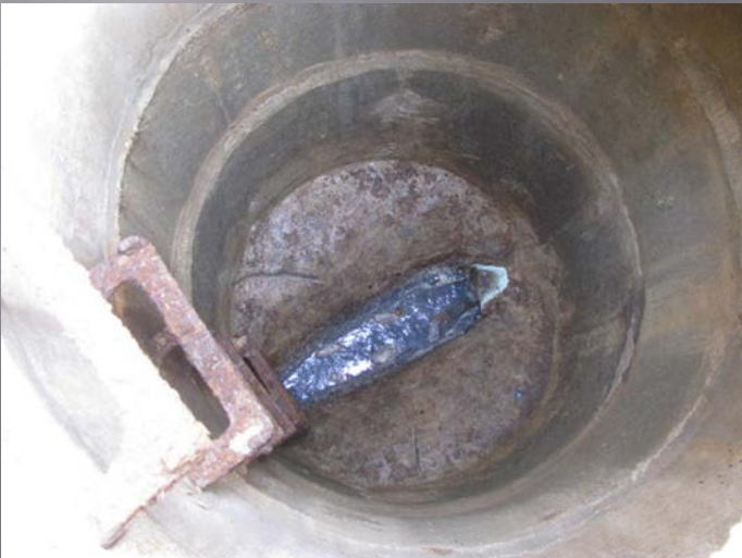
Grease in Manhole outside Chinese restaurant prior to bioaugmentation
